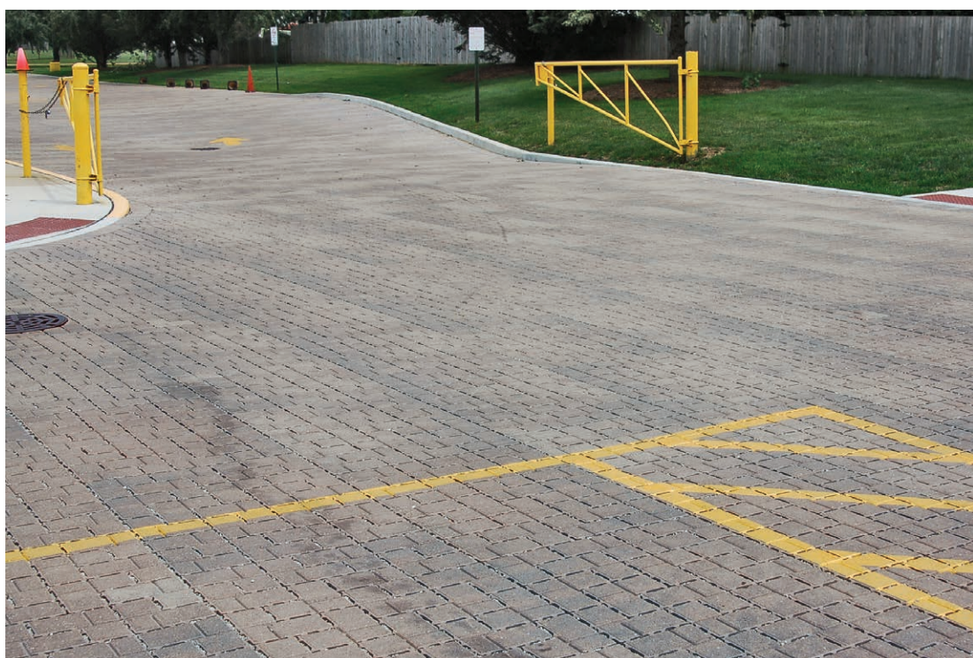
Permeable pavements at Jay Stream Middle School in Carol Stream, Illinois.
