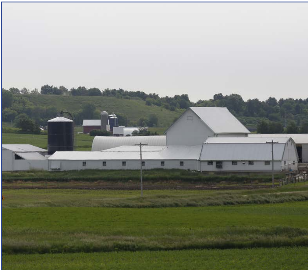
Zeigler Dairy Farms across from EnTech Solutions transports manure via pipeline to the digester
