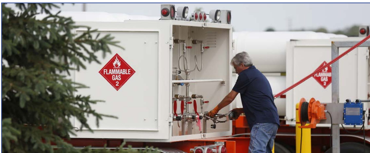
RNG transfer to truck for transport to pipeline injection point, EnTech Solutions, Town of Springfield, WI
